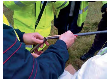
3. The earth line is locked to the hardened steel tip with the leading rod.
