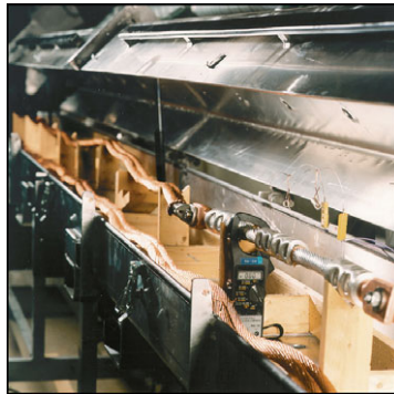
Test of terminals.
